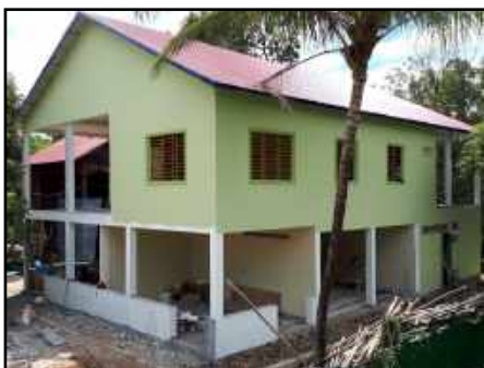
Front view—dorm rooms upstairs, classrooms downstairs.
